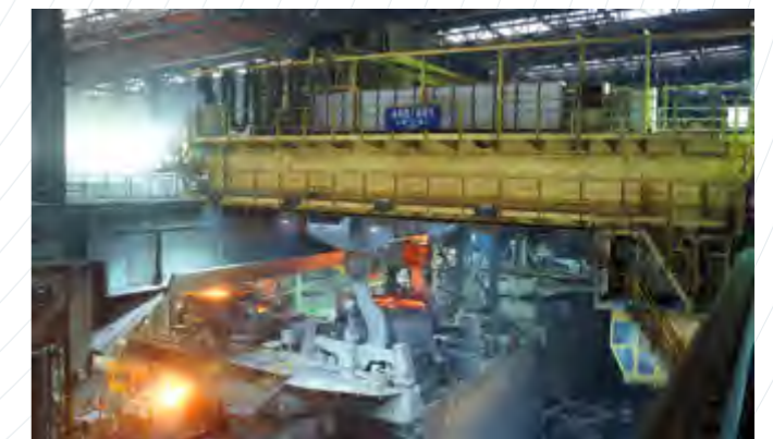
460t铸造起重机 460t Teeming Crane
