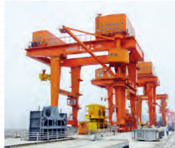
坝顶门式起重机群 Gantry Cranes on Dam Crest
