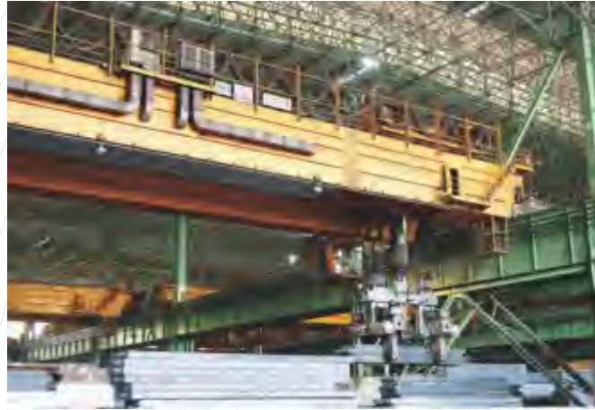
98t板坯夹钳起重机 98t Slab Tong Crane
